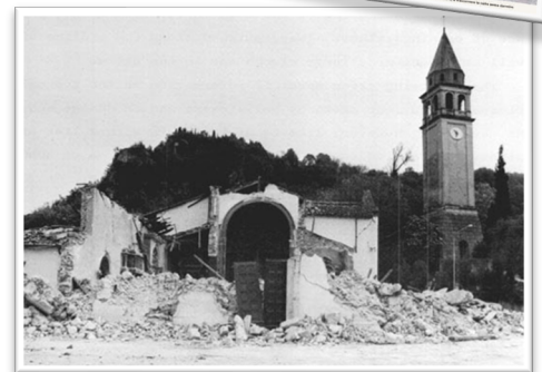
The parish church of Osoppo after the May 6 earthquake. The Bell tower collapsed in the September 15 earthquake.
