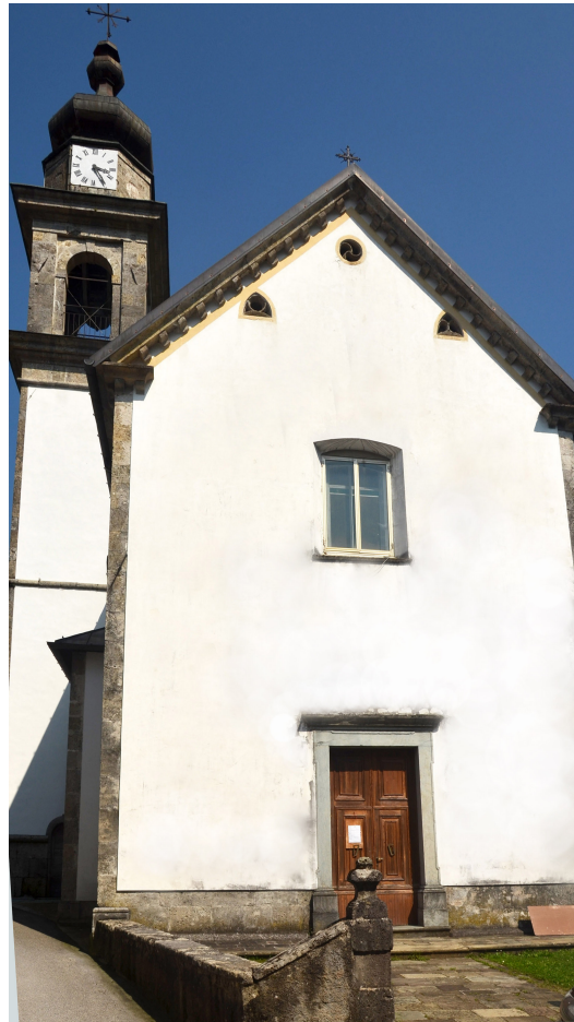
The façade shows the proportions of the church (height-width) and the campanile with the eastern style top.
