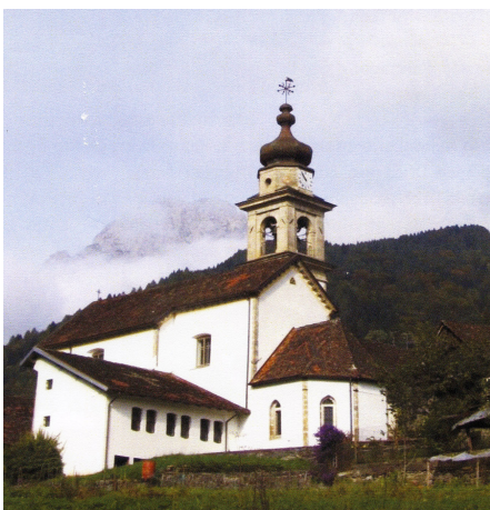
The design features of the building are better shown in this rear view.
